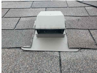
General Images Of Dryer Exhaust Systems:
