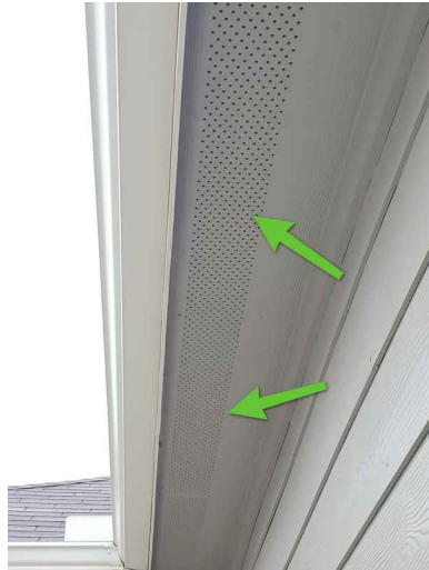
Soffit Vents
