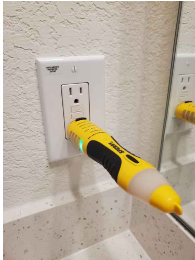
Location Of Laundry Room GFCI Reset : This resets laundry room outlets.
