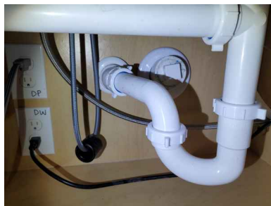
Sewer Cleanout Location: Front
