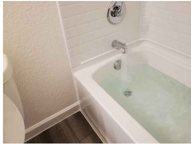
Hall Bathroom Tub
