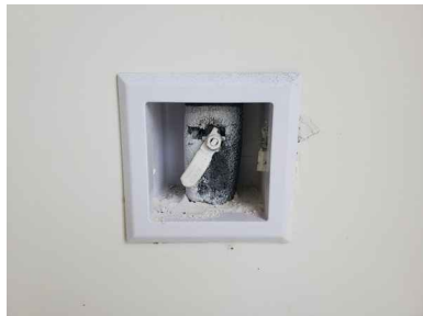
Static Water Pressure Reading: 60-65 PSI
